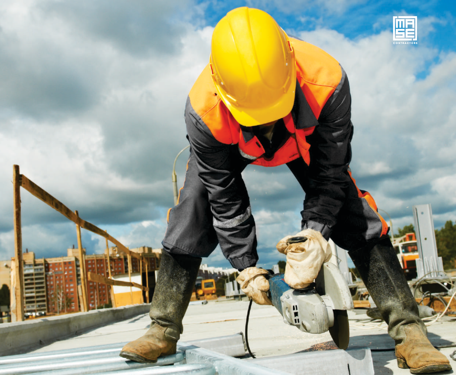
Builder worker with grinder machine cutting metal parts at construction site
